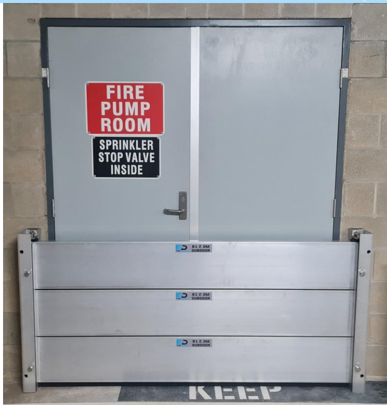
Figure 13 - B1 Sub Doors B1.12(D0.1): FDD0.84x2.0m
