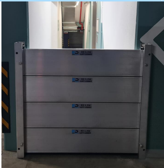
Figure 19 - B3 Lift Lobby B3.05: FDD1.14x1.2m
