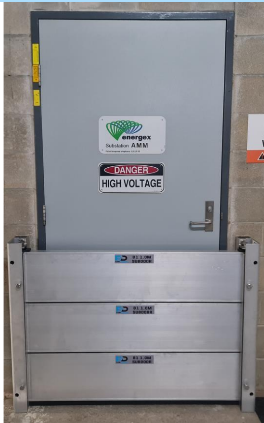
Figure 11 - B1 Sub Doors B1.11(D0.1): FDD0.84x1.0m
