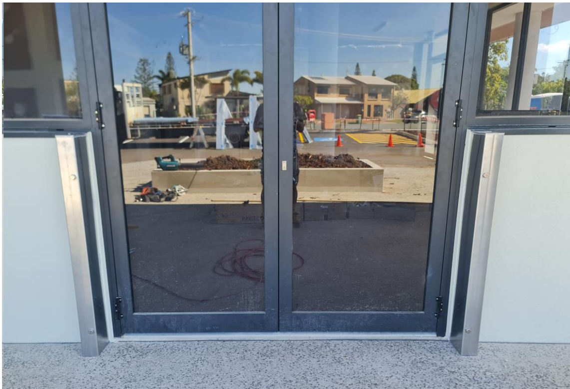
Figure 1 - Typical Flow Defence Demountable Flood Barrier (disassembled)
