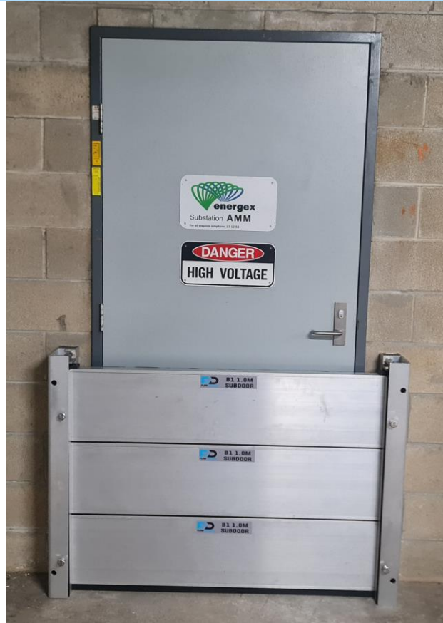
Figure 17 - B1 Sub Doors B1.14(D0.4): FDD0.84x1.0m
