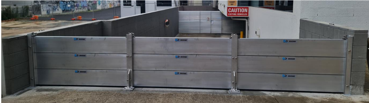
Figure 4 – FDD Driveway/Basement Protection
