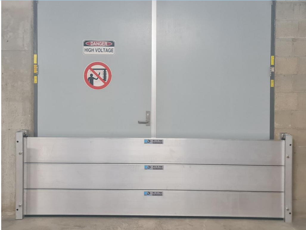
Figure 15 - B1 Sub Doors B1.14(D0.2): FDD0.84x2.7m
