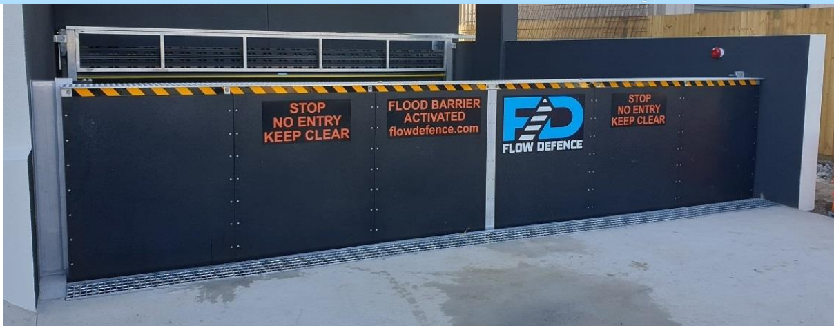
Figure 2 - Typical Flow Defence Hidden Flood Barrier (activated)
