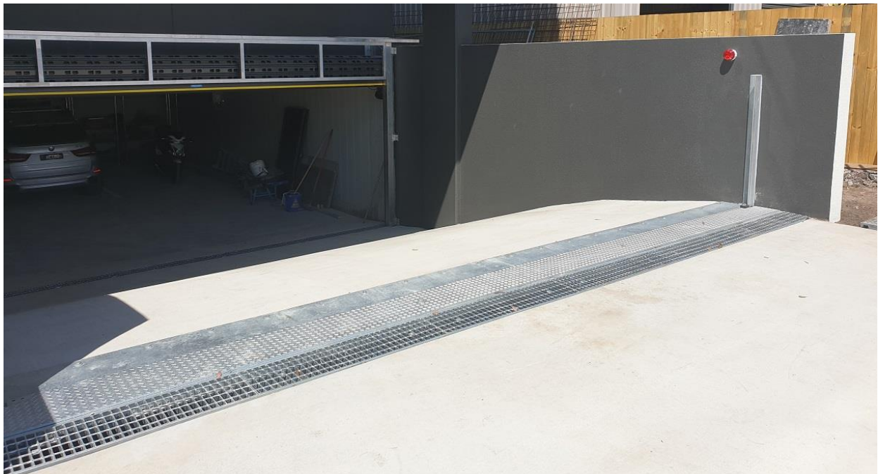
Figure 1 - Typical Flow Defence Hidden Flood Barrier (retracted)
