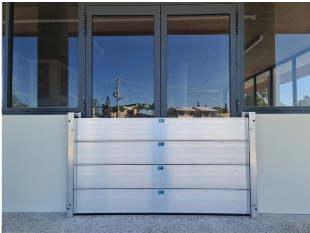
Figure 2 - Typical Flow Defence Demountable Flood Barrier (assembled)
