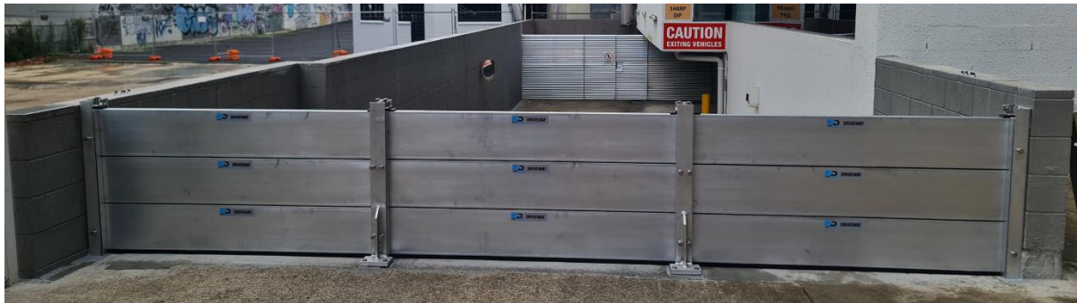
Figure 4 – FDD Driveway/Basement Protection
