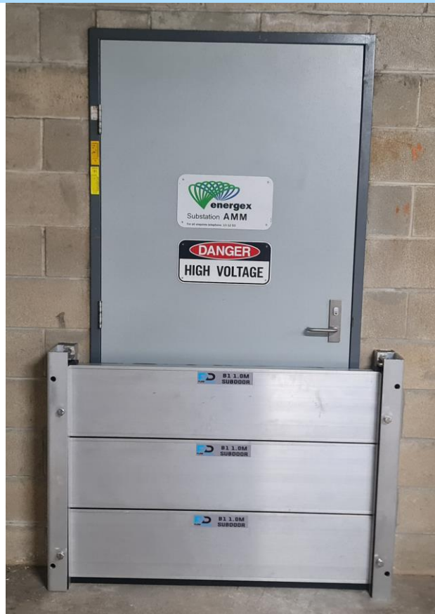
Figure 17 - B1 Sub Doors B1.14(D0.4): FDD0.84x1.0m
