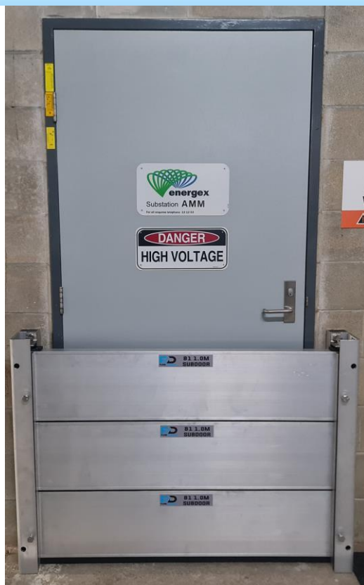
Figure 11 - B1 Sub Doors B1.11(D0.1): FDD0.84x1.0m
