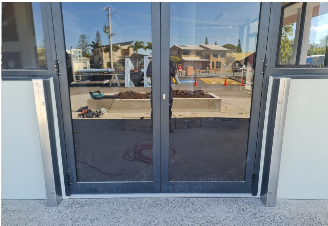
Figure 1 - Typical Flow Defence Demountable Flood Barrier (disassembled)
