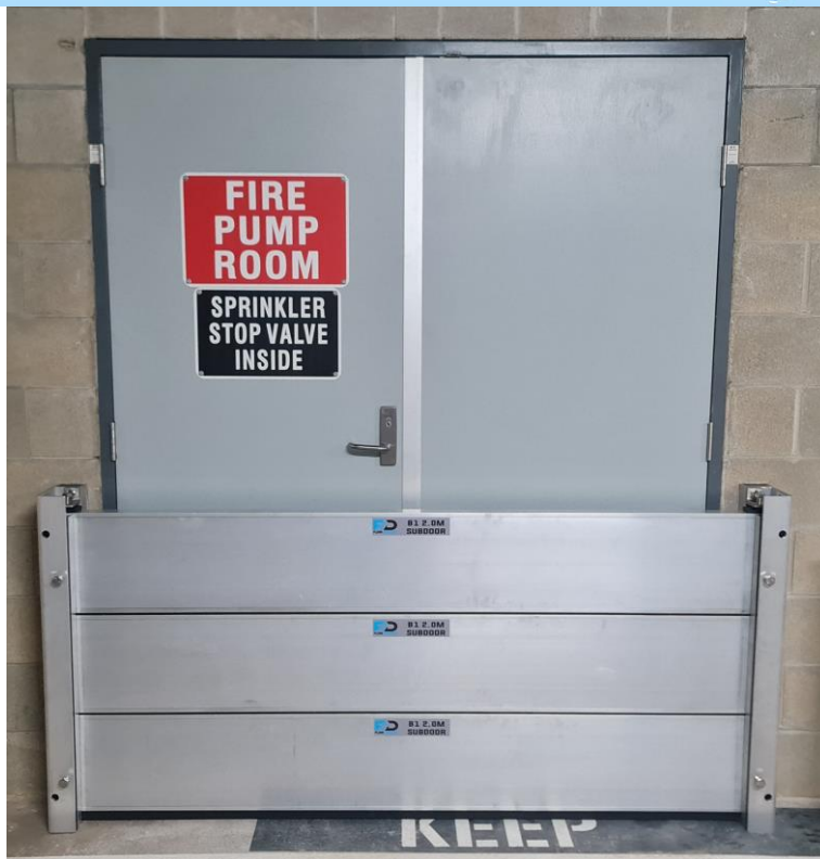
Figure 13 - B1 Sub Doors B1.12(D0.1): FDD0.84x2.0m
