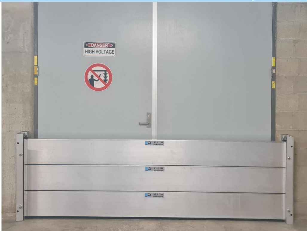
Figure 15 - B1 Sub Doors B1.14(D0.2): FDD0.84x2.7m
