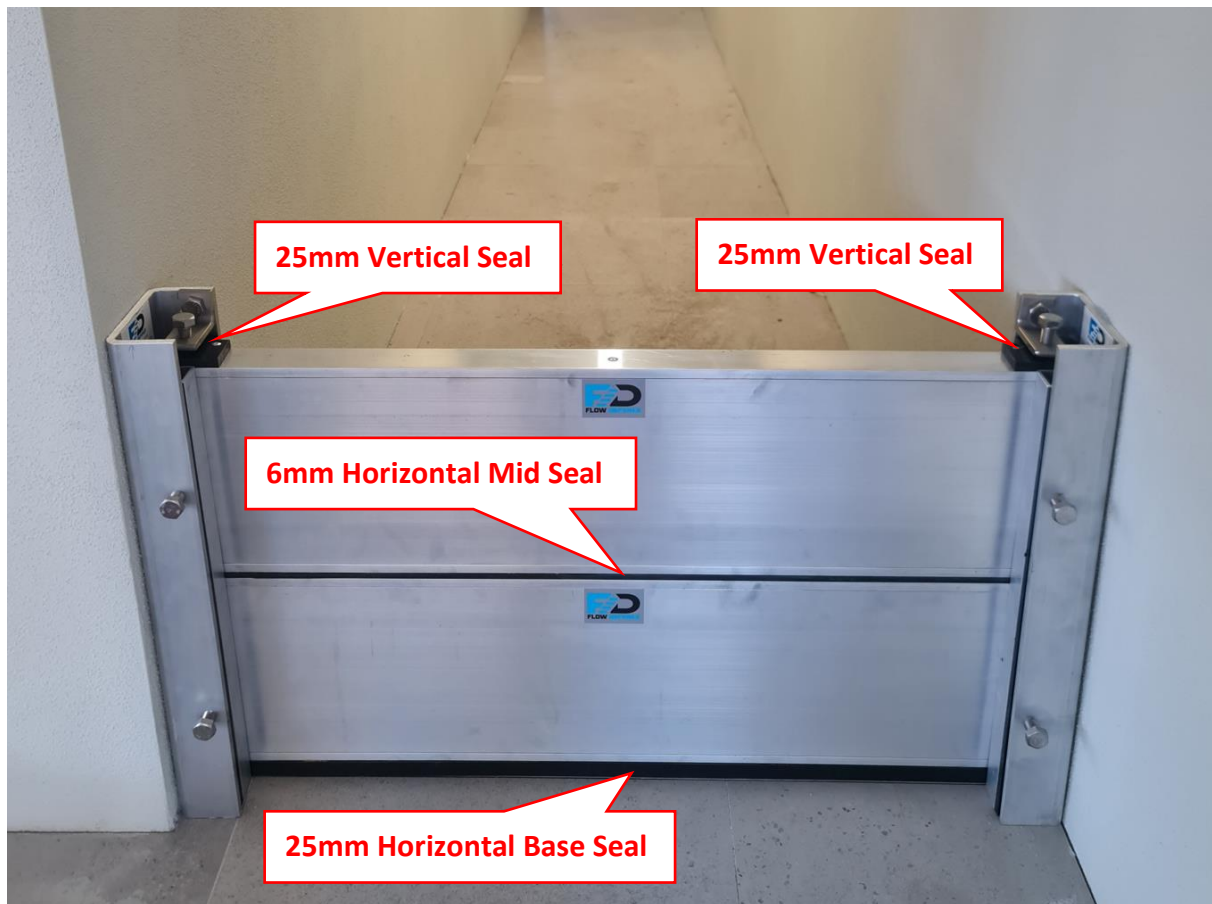
Figure 6 - FDD Sealing Mechanism
