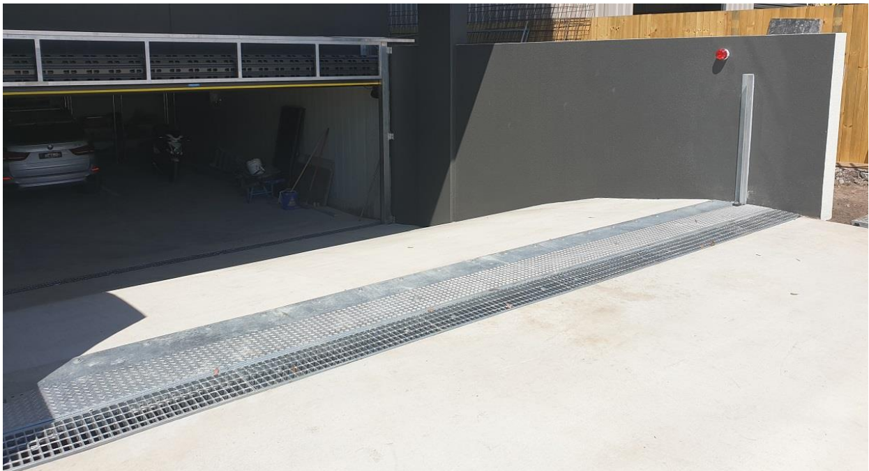
Figure 1 - Typical Flow Defence Hidden Flood Barrier (retracted)
