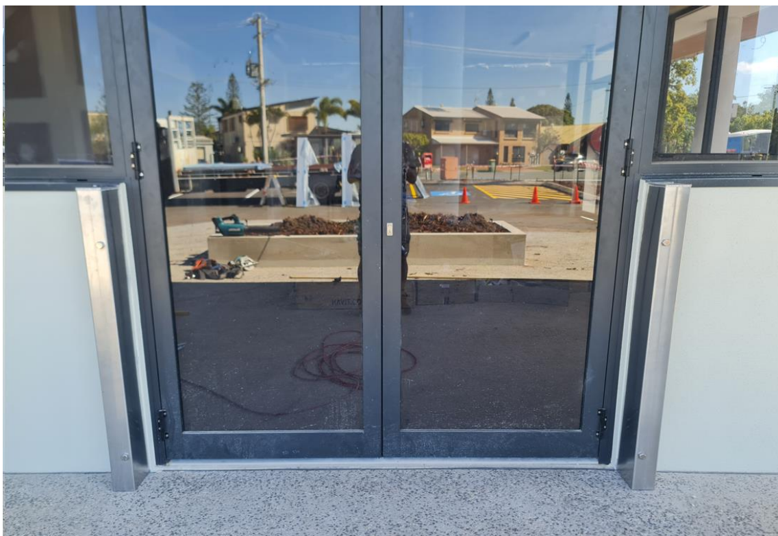
Figure 1 - Typical Flow Defence Demountable Flood Barrier (disassembled)
