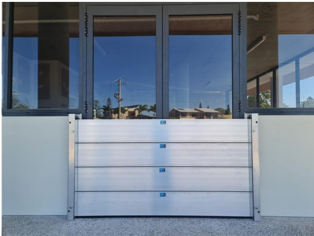
Figure 2 - Typical Flow Defence Demountable Flood Barrier (assembled)
